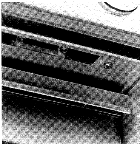
Proper location of water pan.
